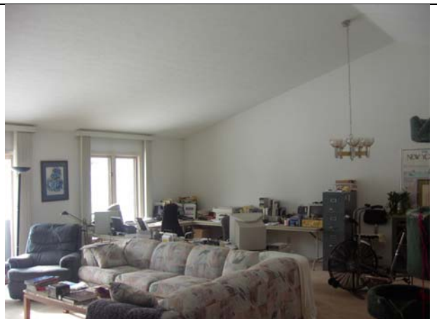
Cathedral locations were not accessible at the inspection time. Conditions at these areas are unknown.
