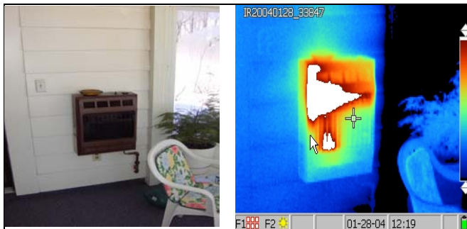
The patio has a ventless heater. The by-product of this is H 2 O and vapor. This unit continually produces humidity when on. The room is used for plants and smoking. Everytime the patio door is opened grains of moisture escape into the dwelling.
